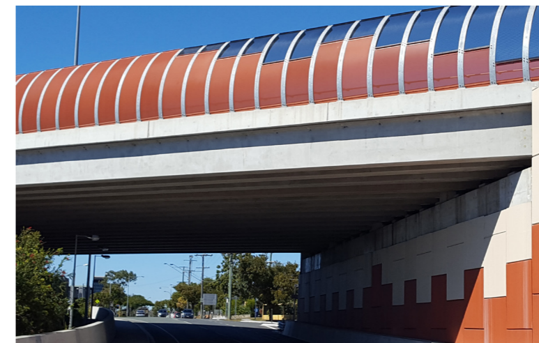
Geebung Overpass - Queensland.
