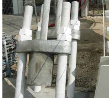
Cable fixing (Paris - France)
