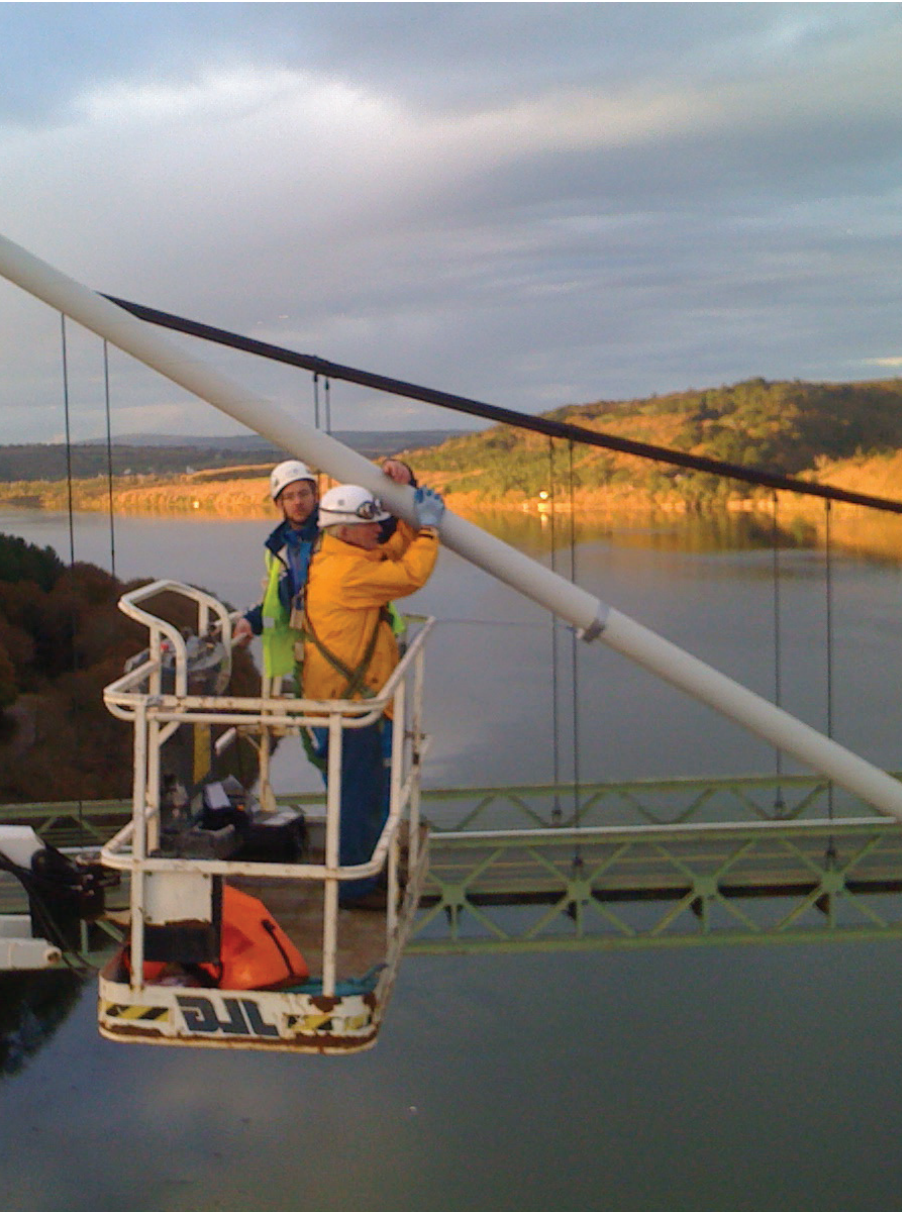
Visual inspection of stay cables
