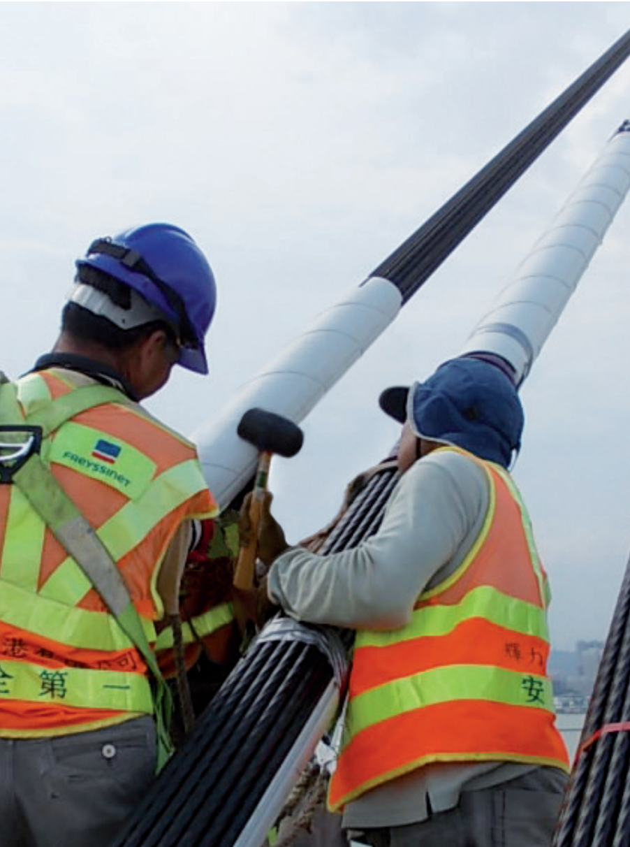
Installation of aerodynamic sheaths on existing stay cables
