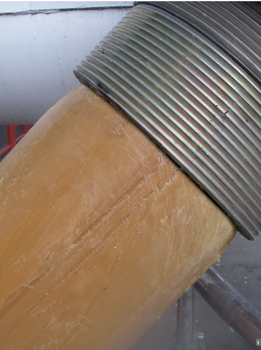
Opening of anchor covers for inspection
