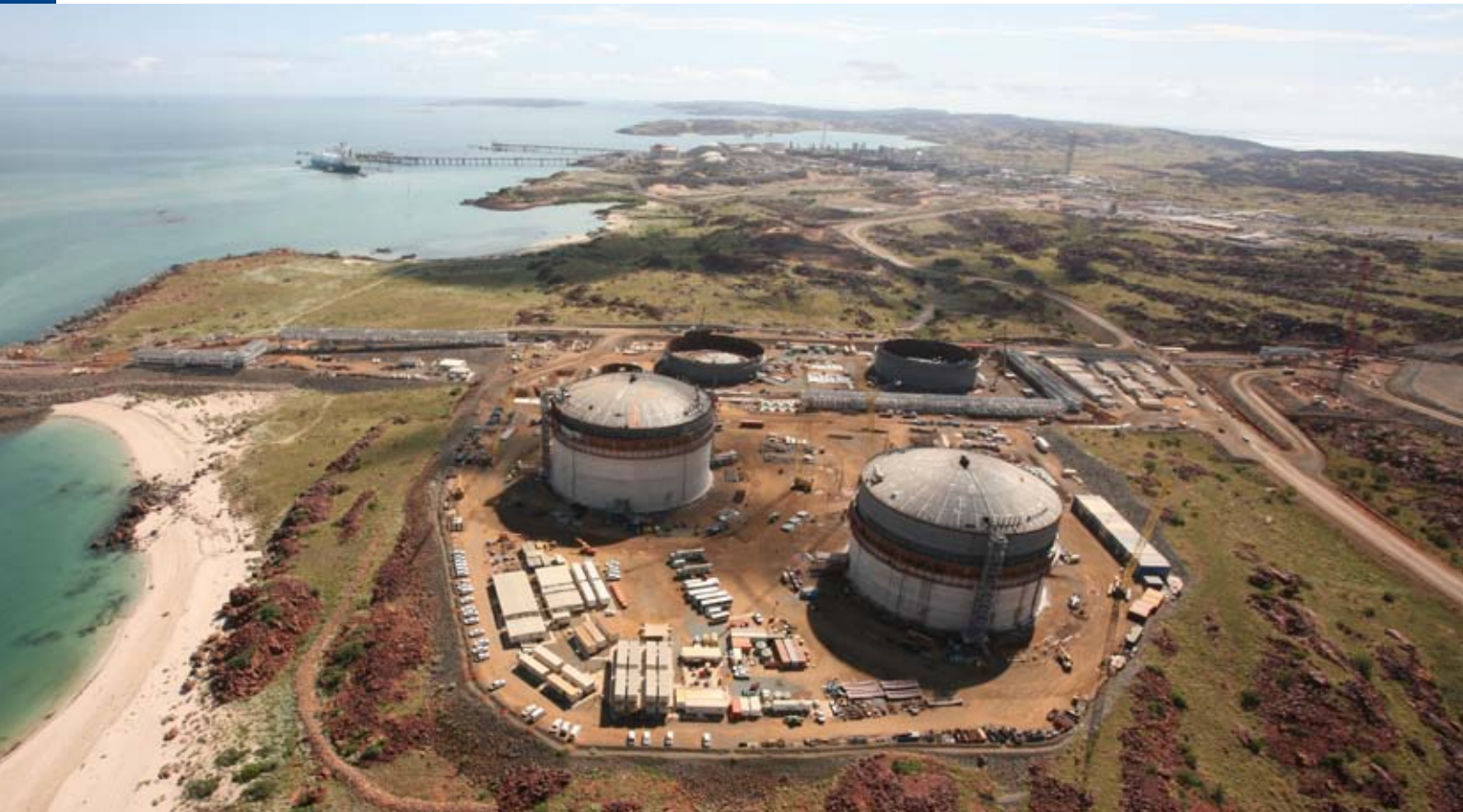
Pluto, Australia, 2 tanks of 120,000 m 3
