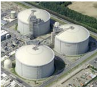
Sakai LNG, Japan, 3 tanks of 140,000 m 3
